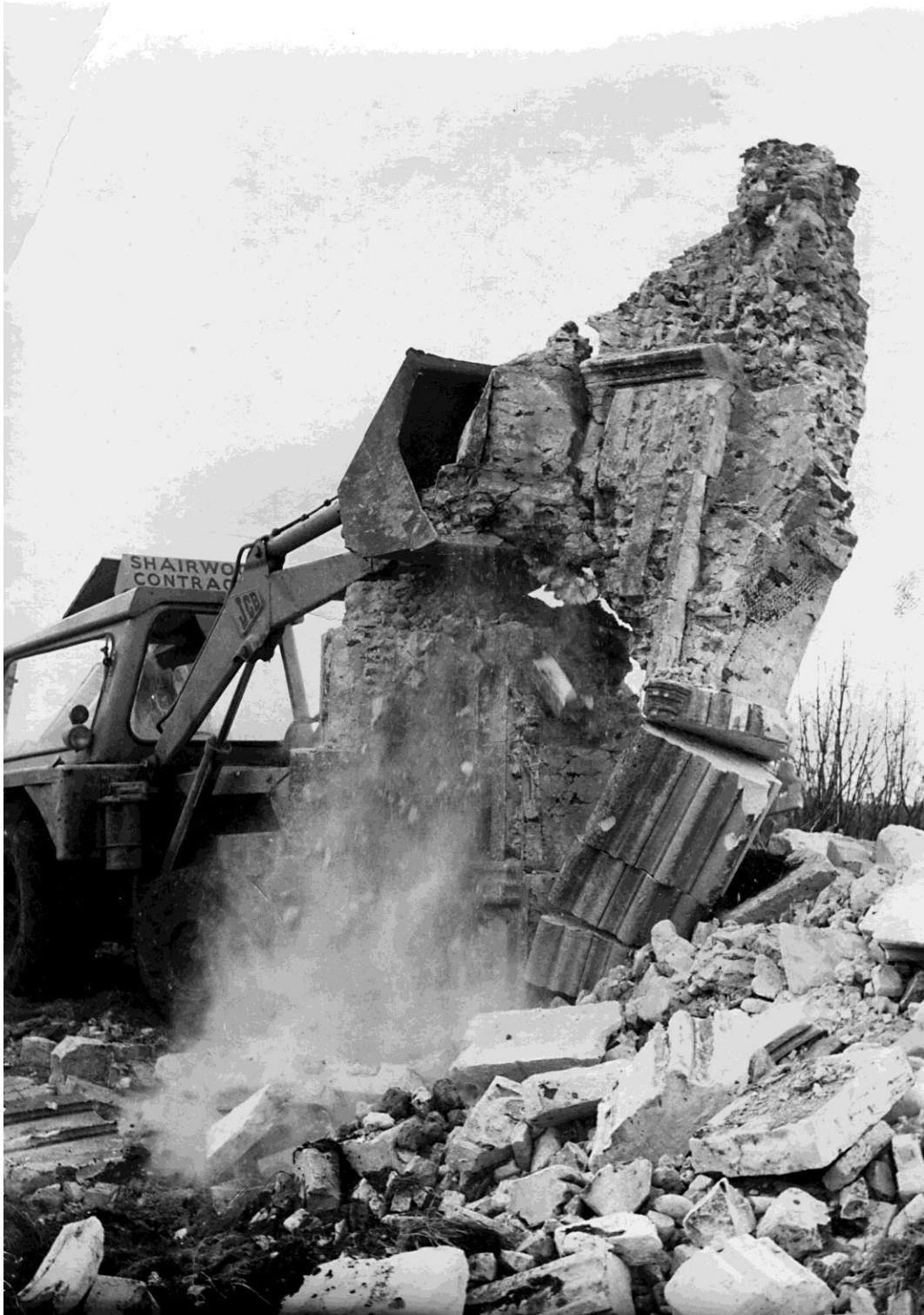
Demolition of the remains of Mistley (Heath) Church
